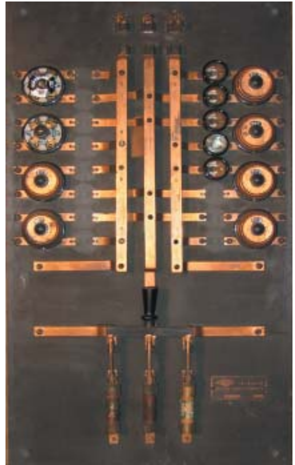
State-of-the-art circuit protection and distribution panel board from circa 1920. Bare copper bars were bolted to a 1-inch machined slate base, with rotary switches and plug fuses. Weight: 60 lb!
